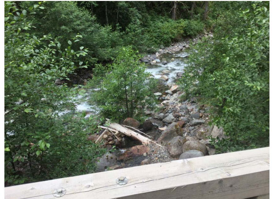
Looking downstream from deck
