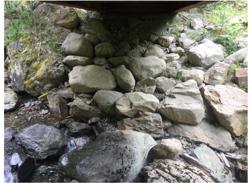
Left Bank Abutment when facing downstream
