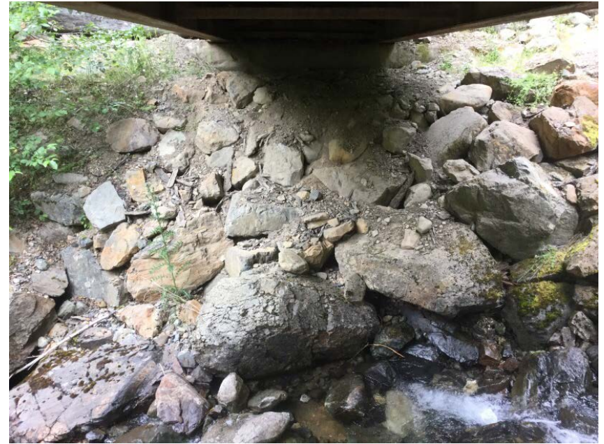
Right Bank Abutment when facing downstream
